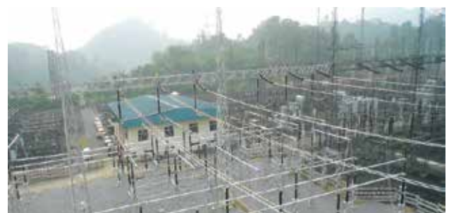
Mambong and Entinggan 275kV substation project
