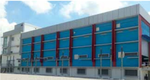
Financial Centre 132/33kV GIS Substation
