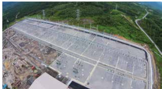
Murum Junction 275/33kV substation
