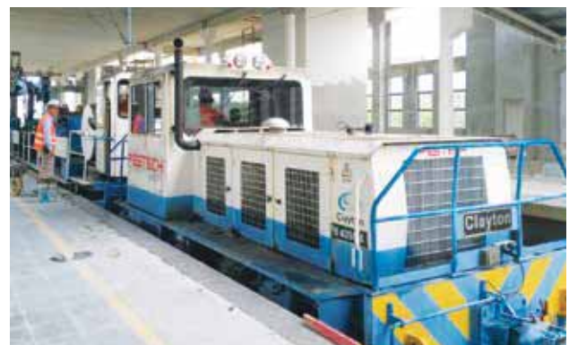
Subang Skypark Double Track Electrification Project
