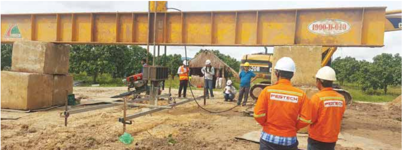
Foundation uplift test for 500kV SHV Project
