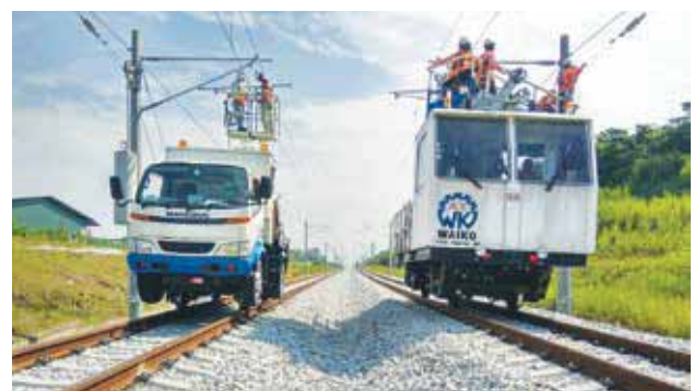
KTM Rehabilitation Project
