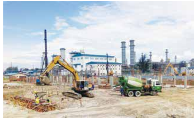
Overall view of new Bintulu B, 275/132kV substation establishment project.
