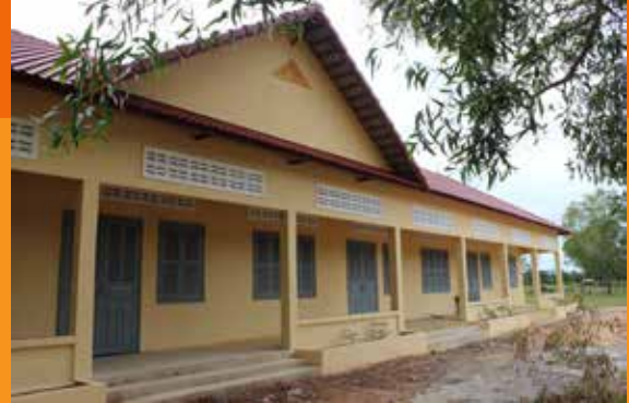
Built 5 classrooms for Student at Pursat Province, Cambodia
