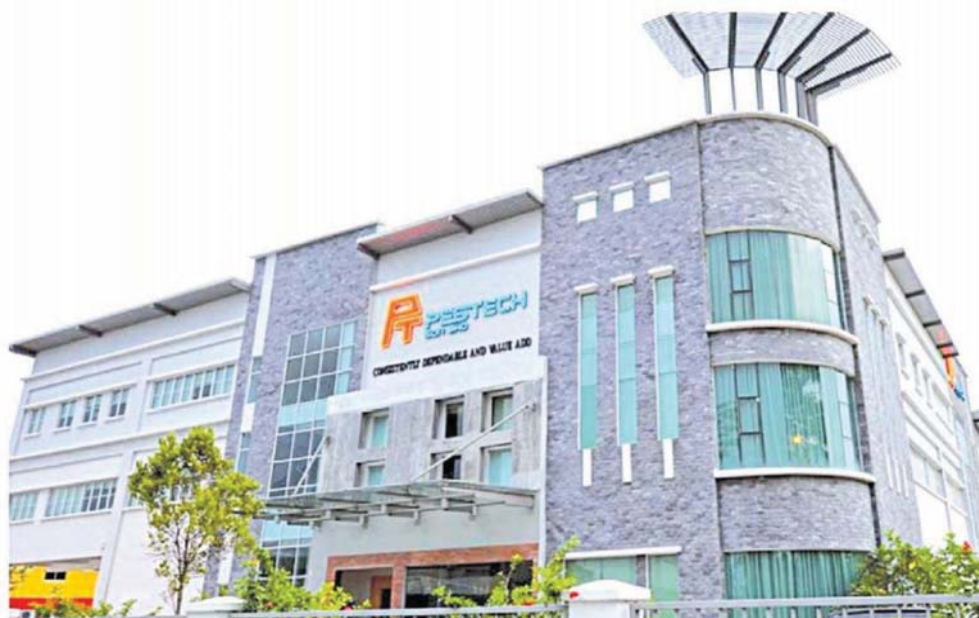
Pestech's latest contract win from NGCP has garnered positive views given that this is another major power infrastructure project awarded by the latter.
